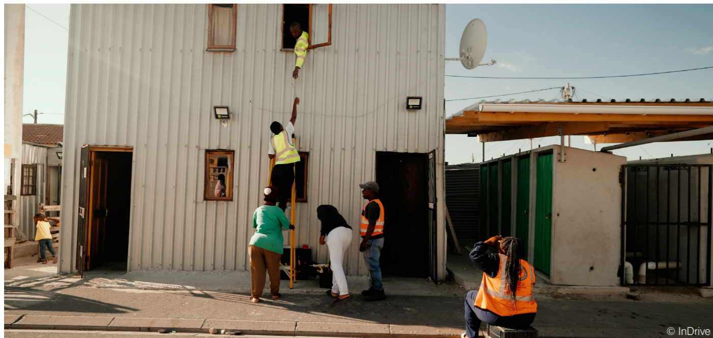
Local team installs lights, empowering residents to manage their own safety
