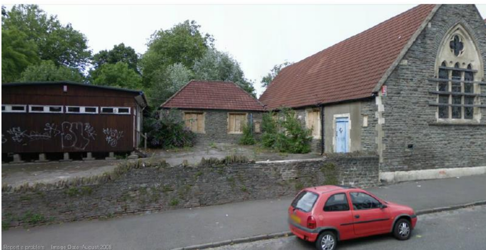
325 Fishpond Road before development (Bristol CLT, n.d.)
